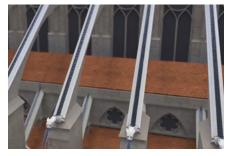
**RAINWATER MANAGEMENT**. The cathedral's rainwater drainage system must handle some 23,000 liters in an average downpour. During a major storm, the weight to be borne is colossal, since the roof area is immense. Without the ingenuity of the builders of Notre-Dame, it would have collapsed long ago. How did they achieve this? The ingenious system of gutters and gargoyles they designed has survived until now, with barely any modifications.
