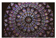
**STANDARDIZATION.** Early on, the builders realized that the standardization of stone blocks made it possible to increase productivity. The rosettes are a perfect example to illustrate this. Just observe the rosettes to demonstrate. The symmetrical repetition of the same patterns, initially drawn, limits the variety of stone templates to produce.
