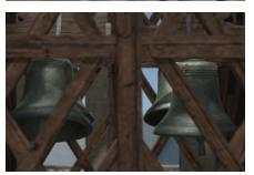
**THE BELLS.** How does one ring a bell like Emmanuel, weighing 14 tonnes, without bringing the whole tower down? The key to this is the belfry, the wooden structure which does not touch the walls of the tower but which just rests on four stone slabs, absorbing the vibrations.
