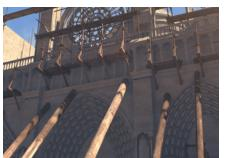
**THE TILT**. Notre-Dame de Paris nearly became the French equivalent of the leaning tower of Pisa. Its façade leans forwards by 30 centimeters — visible by the naked eye, once one knows to look. The builders had to wait for the block leaning forward to stabilize before they built on upwards, this time vertically.
